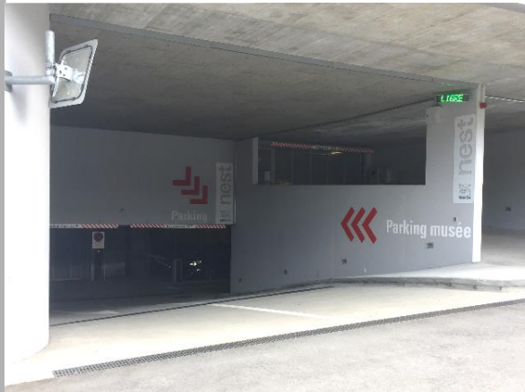
The nest parking is located on the low level of the Rue des Bosquets
